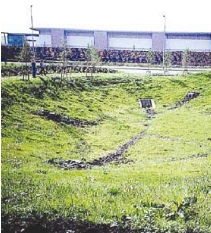
(a) Detention basin fitted in the centre of a motorway roundabout
