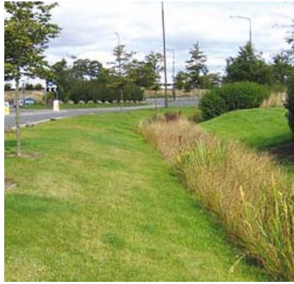
(b) Swales and basins can be incorporated as landscaped features where they would be looked after as part of the normal maintenance contract. Swales may conduct water to other features whilst also providing some infiltration.
