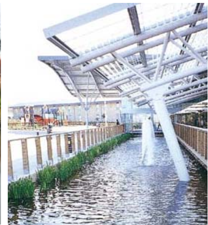
(c) Roof water is directed into this storage pond which serves as an attractive feature of Wheatley Services Area on the M40
