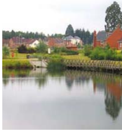
(b) Ponds and wetlands are typically fitted as the final stage of a SUDS system for a major development
