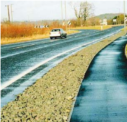
(a) Infiltration trench alongside a road – no kerbs or gullies needed to be incorporated in the design
