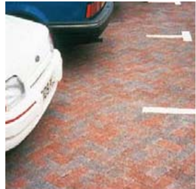
(c) Pervious pavement reduces the risk of surface runoff flooding without compromising on the car park's utility
