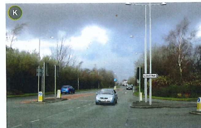
View K - View north highlighting Chain House Lane and Penwortham Way junction.
