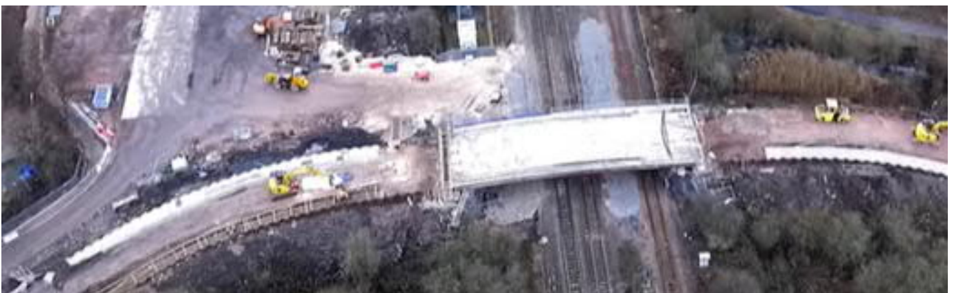
Awsworth Road Bridge, Ilkeston, steel composite 33m single span (7.65m carriageway & 2m footpath) on existing foundations – (2017) - c£3m
