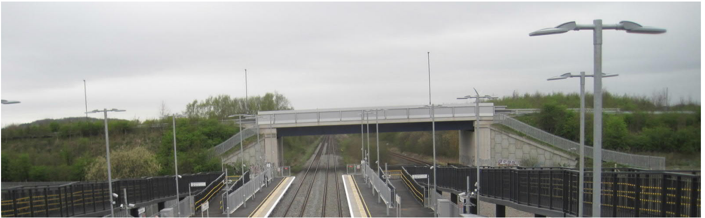
Ilkeston Station Footbridge, 37m single span (3m wide footbridge) – (2017) - c£2.5m
