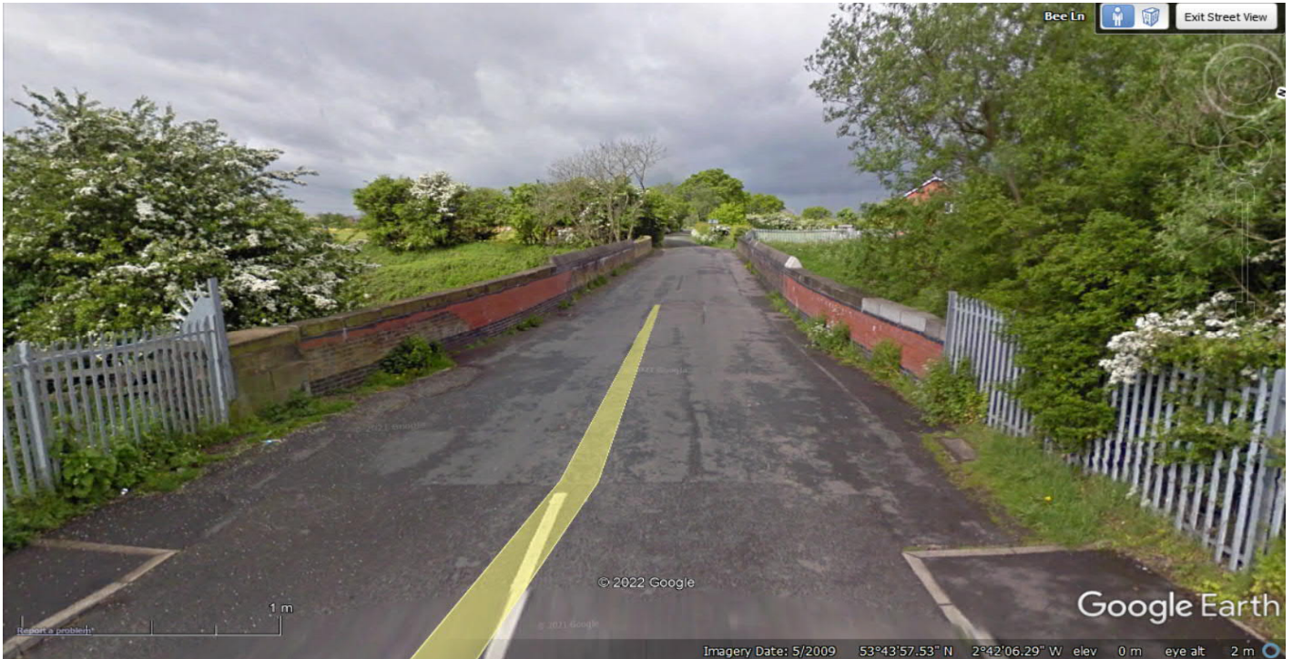
Figure 4 - Bee Lane Bridge (looking West)
