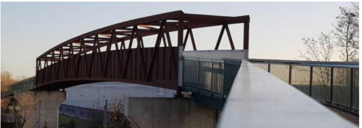
Awsworth Road Bridge, Ilkeston, steel composite 33m single span (7.65m carriageway & 2m footpath) on existing foundations – (2017) - c£3m
