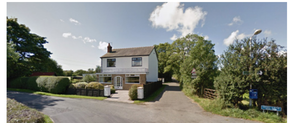
Existing Area Character Mature and rich hedgerows along Bee Lane, a housing sample on Bee Lane plus, an existing mature feature Oak Tree. The Lanes, Penwortham | Landscape Strategy24
