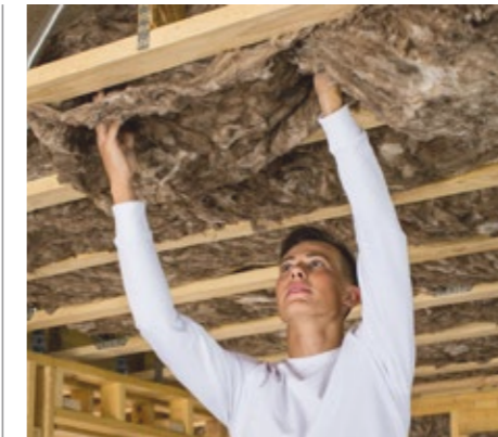
Fabric improvements and appropriate insulation
