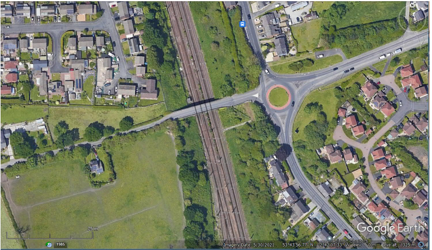
Figure 2 - Bee Lane Bridge
