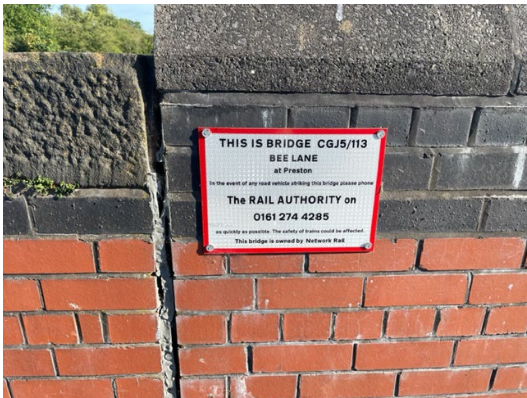
Photo 7: Bee Lane Bridge is owned by Network Rail.
