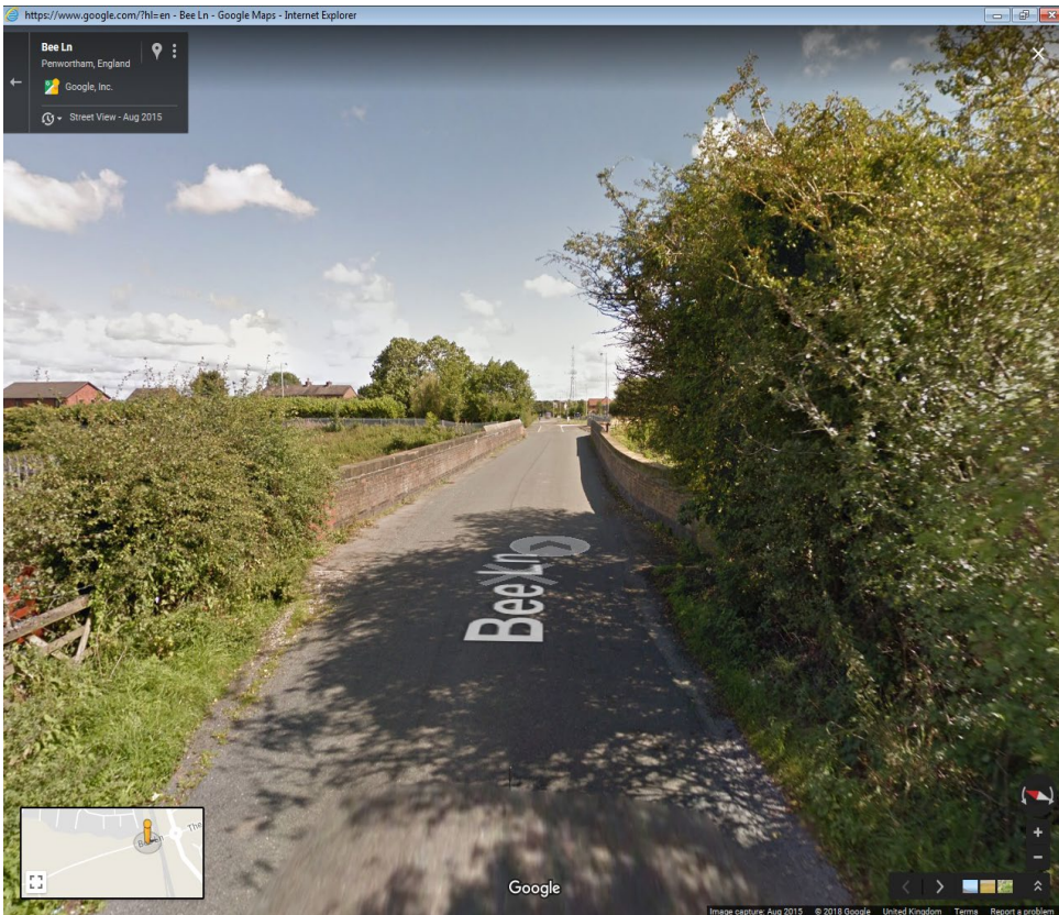
Photo 5: Bee Lane Bridge. No separation of users and no protection of parapets. Parapet walls are low.
