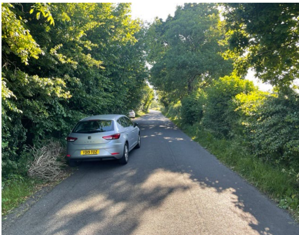
Photo 8: Bee Lane with Vehicle. Limited width for passing vehicles and scope for conflict with pedestrians and cyclists. Note vehicle is off the carriageway to enable sufficient passing space.
