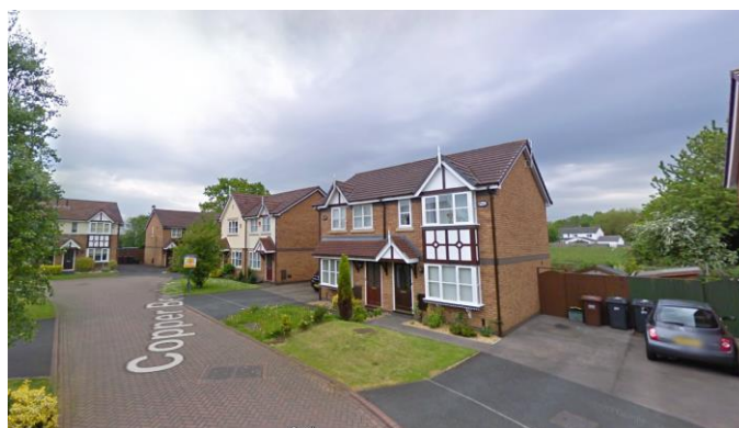
Figure 22 – Extract from Google Earth of Copper Beeches
