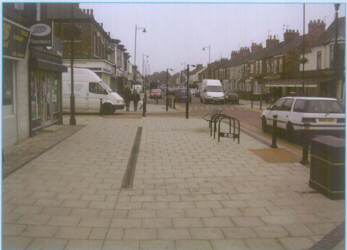
Footways widened significantly by narrowing carriageway
