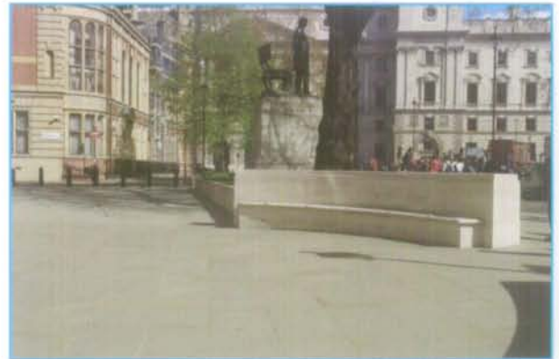
Anti-ram walls that also provide seating outside the Supreme Court, Parliament Square
