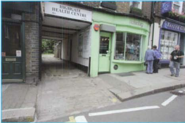
Footway crossover access to commercial premises
