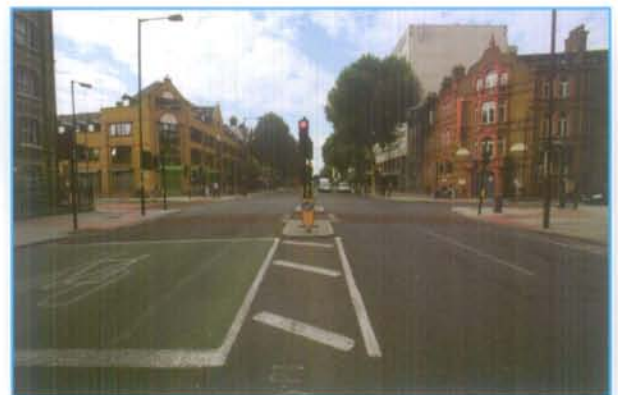
Traffic signal junction with clear and simple pedestrian crossings and advance cycle stop lines. Note lack of guardrailling and buildings close to junction corner, and tight corner radii.
