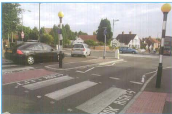
Zebra crossing close to mini-roundabout exit.
