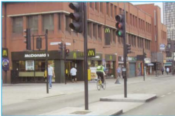
Pedestrian refuge without keep left bollards, Walworth Road Mixed Priority Route scheme
