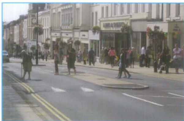
These simple pedestrian refuges were provided on The Parade, Leamington Spa MPR project. Note the absence of keep left bollards, but also the intrusive road markings.
