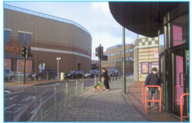
Segregated left turn lanes make pedestrian crossing movements more complex and slow, as well as adding to clutter.
