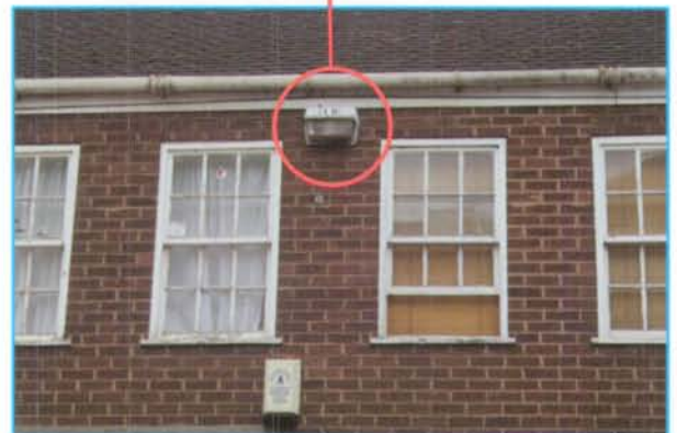
Inconspicuous lighting units on buildings help to minimise clutter in this village high street.
