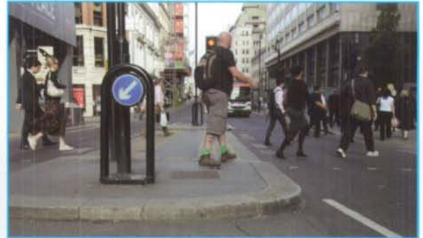
Sign to diagram 610 mounted on hoop top frame.
