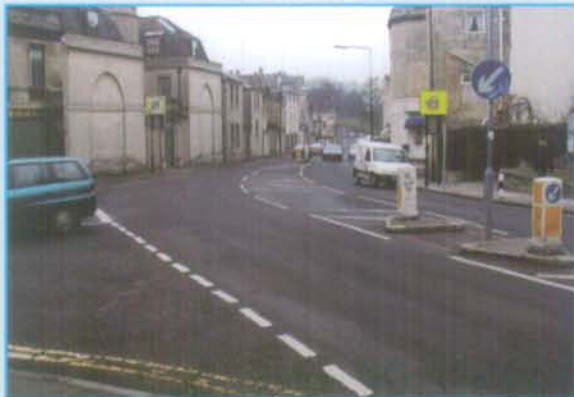
Julian Road Bath – Before and After
