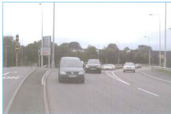
Cyclists leaving this roundabout can find themselves in the outside lane of a dual carriageway.
