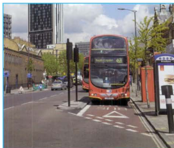
Bus Advance Area, Walworth Road MPR scheme
