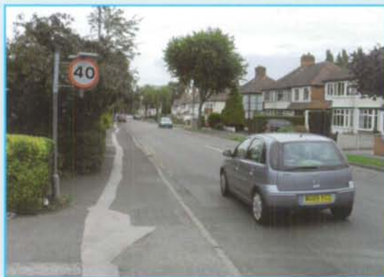
Single Lane, Frontage Access, On-Street Parking
