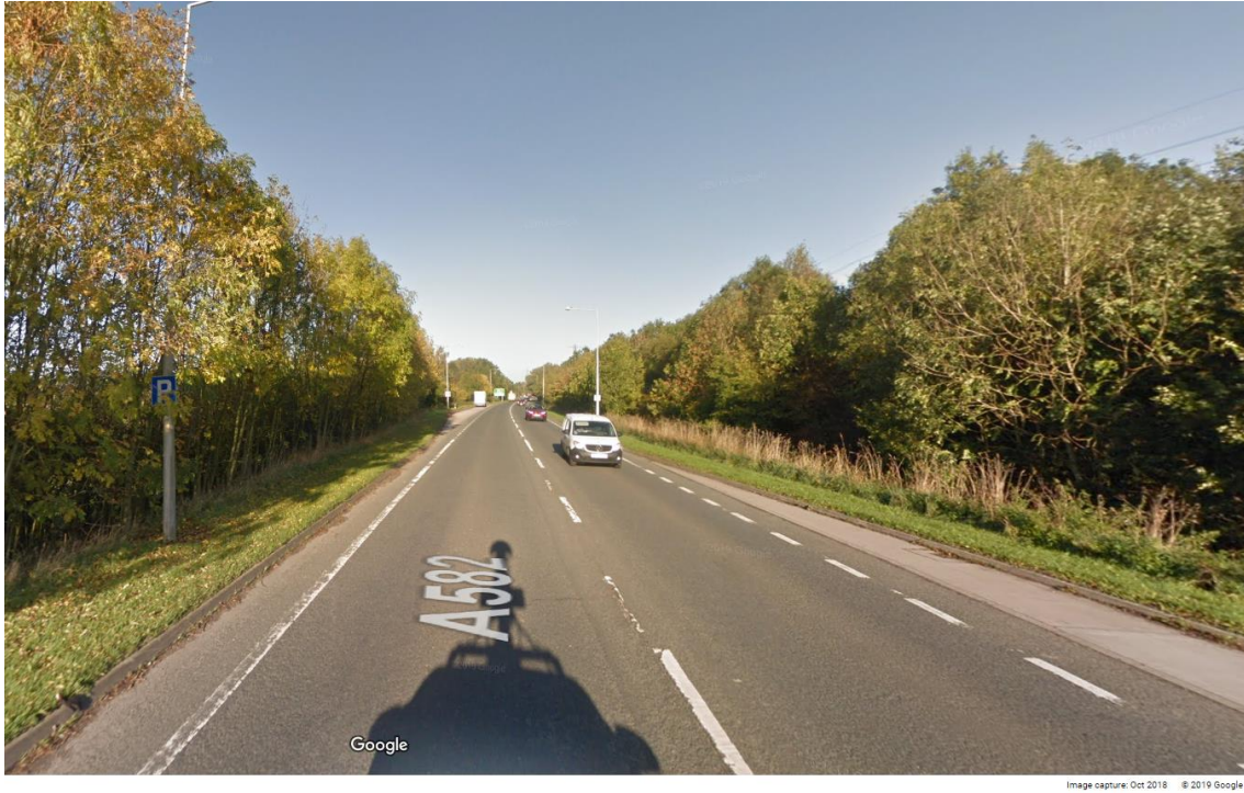
Figure 3.2-R: Street level imagery of A582 Penwortham Way North (Point 4 from Table 3.2-iii/Figure 3.2-G)
