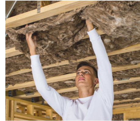
Fabric improvements and appropriate insulation
