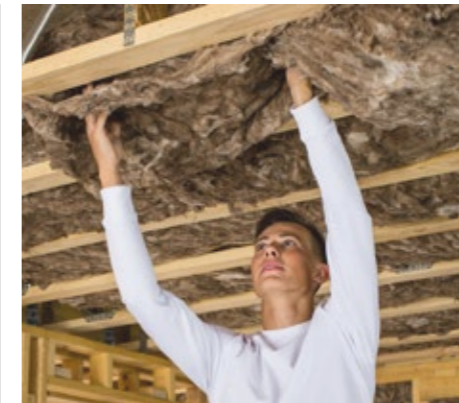
Fabric improvements and appropriate insulation
