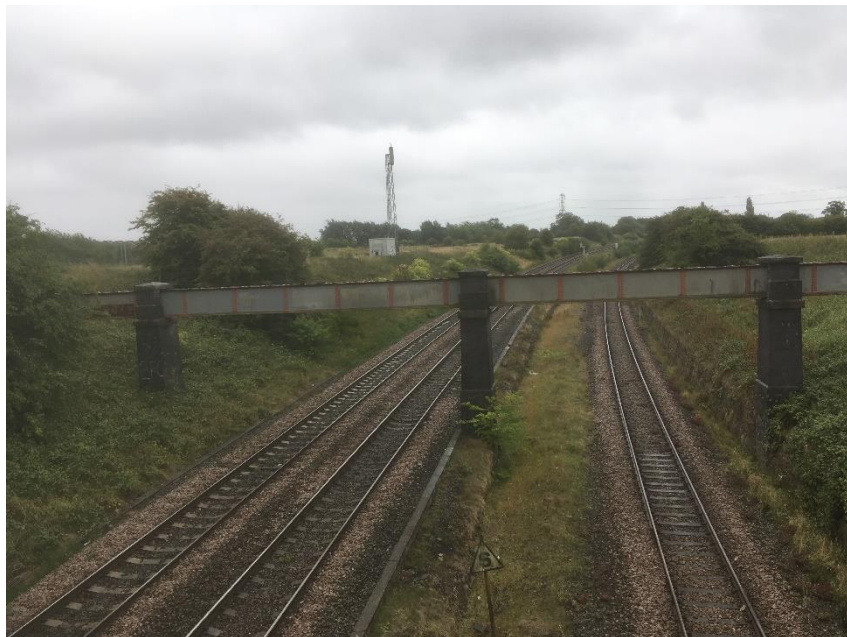
Photo 88: Looking south along railway line on the sites eastern boundary
