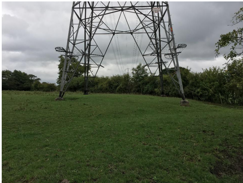
Photo 16: Looking towards pylon in a western field
