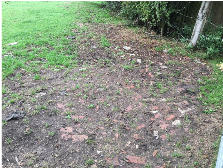
Photo 7: Evidence of fill material around access point to western fields
