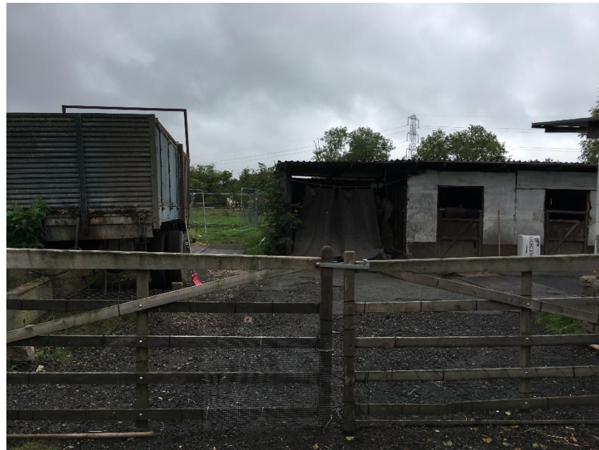
Photo 41: Looking south from Bee Lane towards stables
