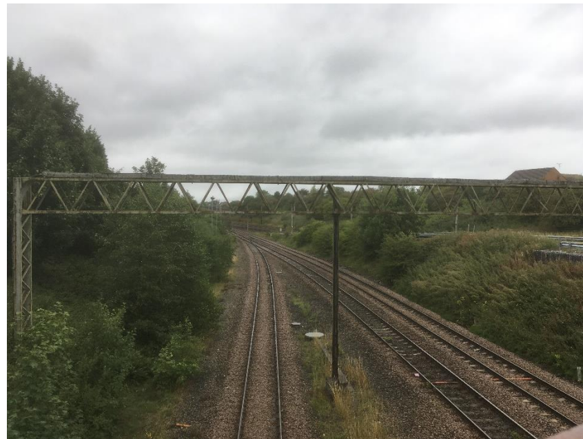
Photo 89: Looking north along railway line on the sites eastern boundary
