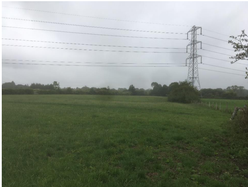
Photo 79: Looking west across central field bounding safeguarded land
