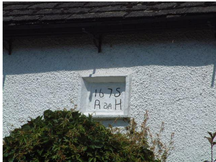
Yeoman's House date detailing: 1675
